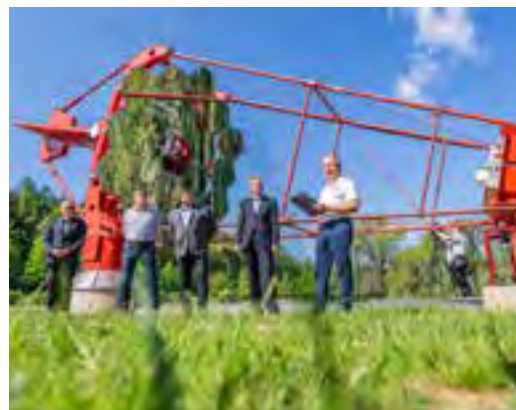
Installation of the Cherenkov telescope in Ondřejov
